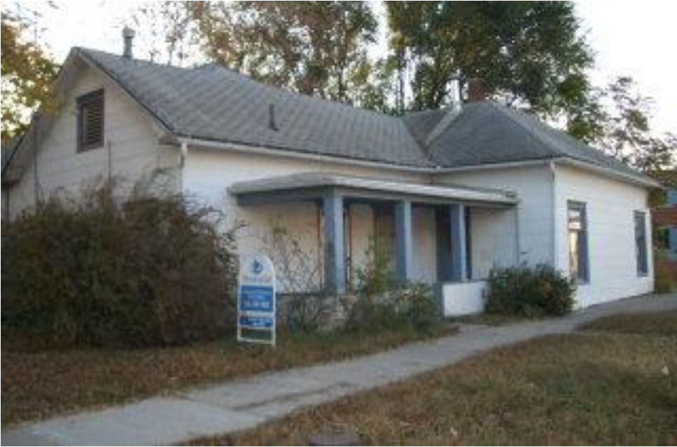
General Repair Needed
